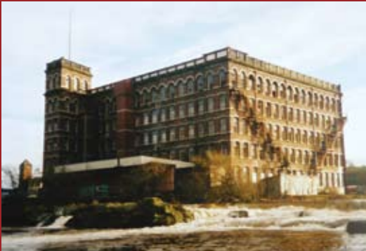
Domestic Finishing Mill, Anchor Mills, Paisley The Anchor Mills complex was founded in 1812. Completed in 1886, the Domestic Finishing Mill had a working life of nearly 100 years, finally closing in 1983. As a building, this Category A-listed structure is unusual. It has a primarily red brick exterior supported by cast-iron columns round a central atrium. The complex enjoys a central location in Paisley. Since production ceased, development
